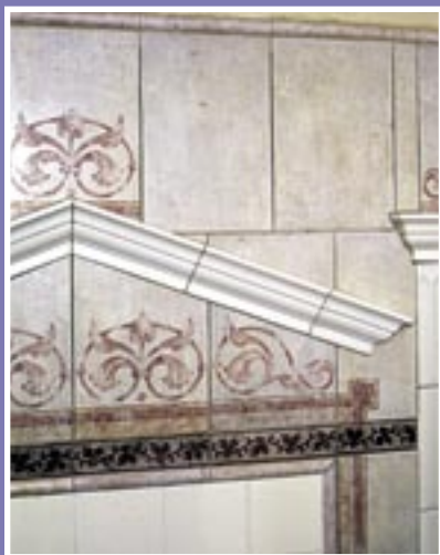
A pediment and column is created using special relief tiles and trims, and the tympanum is filled with fresco motif background tiles.
